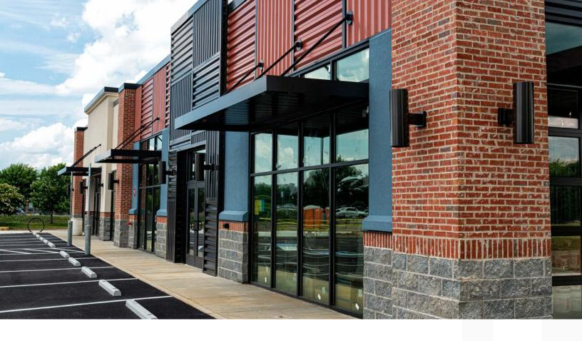
Modern concrete masonry units, like their ancient predecessors, are made from a mix of water, aggregate and cement molded into a sold block as hard as stone and just as resilient. They are designed to exceed required compressive strength.
